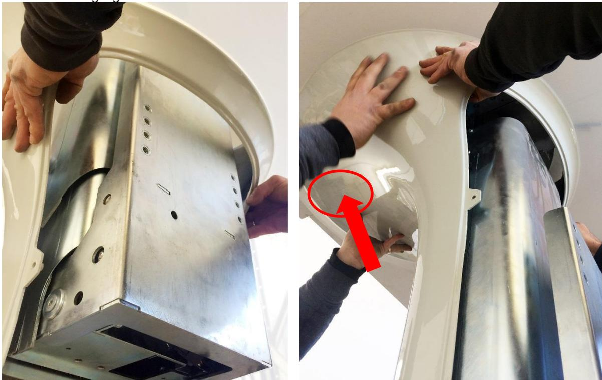
D) Introduce the shell from below, lifting it up to the attachment point of the magnet.
